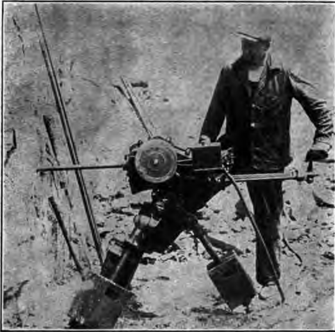
Fig. 43. Scott Drill (C-7) on Drifting Work.
